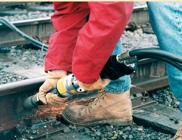
The GR60 Cup Stone Grinder was designed to meet rugged grinding needs while the HG60 Bull Nose Grinder is ideal for grinding and de-burring drilled holes in rail. The HG80 provides an ideal grinding tool from cleaning up a thermite weld to grinding a radius on frogs.
