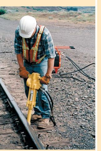
Stanley's SD67 Spike Driver is rugged and lightweight for use in medium to heavy-duty spike driving. The anti-vibration handle and the two length options, help reduce operator fatigue.
